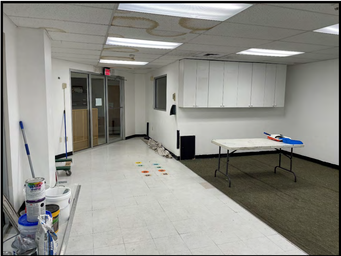
First floor classroom space
