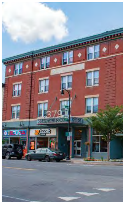
Capitol Square Apartments Pittsfield, MA 69 Units - 71,500 sq ft
