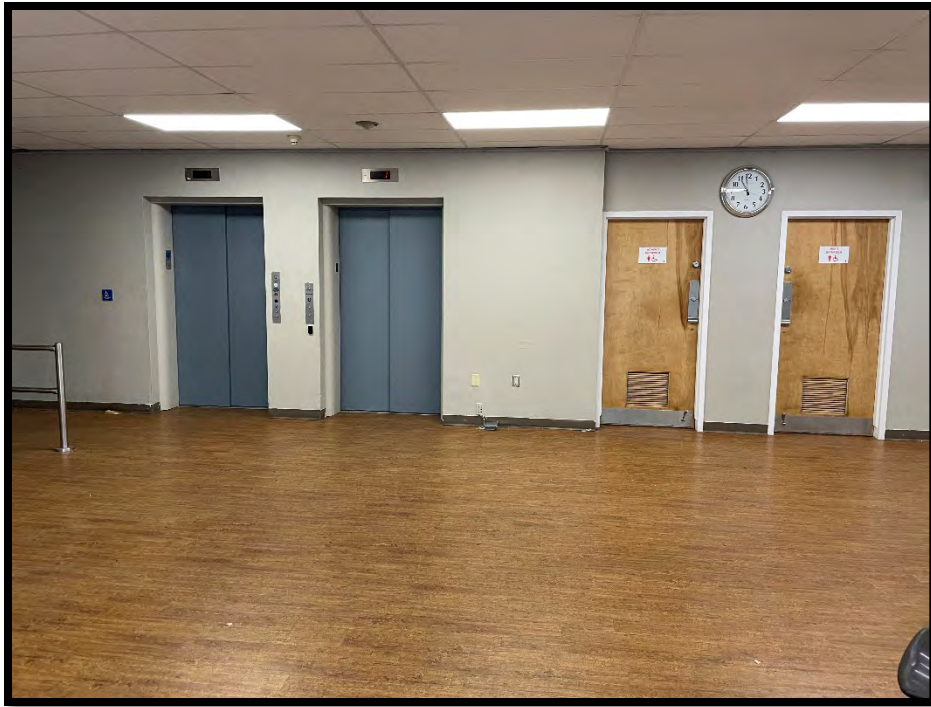
Former main lobby
